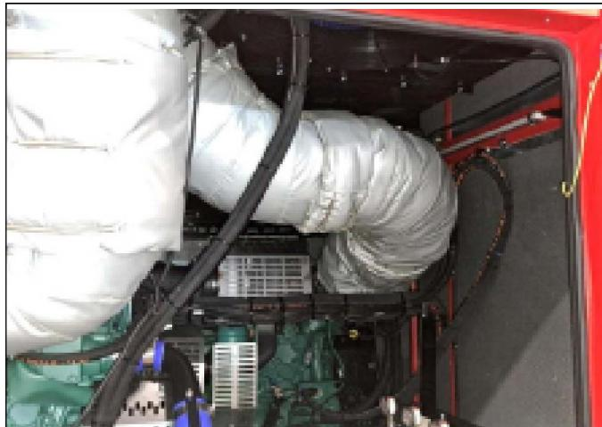
Figure 1-60. Water Discharge Duct Locations
