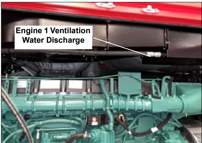
Figure 1-59. Discharge Duct
