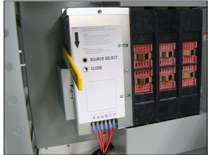
Figure 18. ATS Manual Operating Handle in Use.
