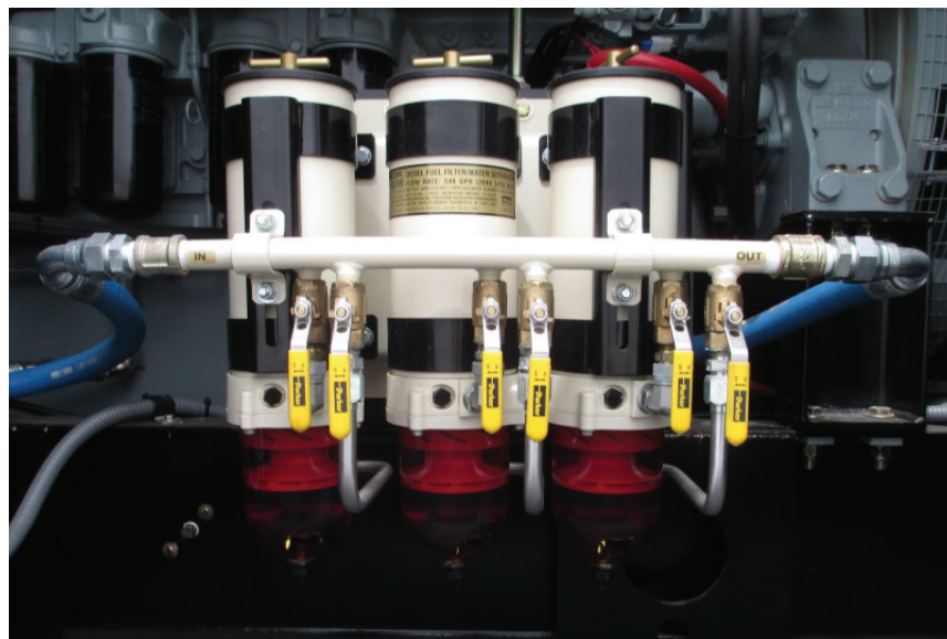
Figure 21 - Fuel/Water Separators
