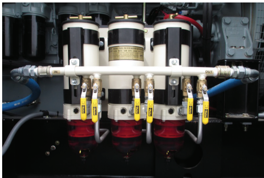
Figure 9 - Fuel/Water Separators
